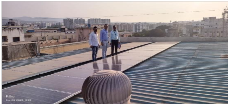
Energy efficient fan and solar roof top
